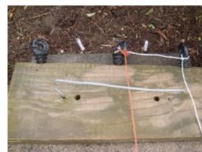
The energiser is in our garage, which has a window in the top of the door into the house passage, so as we pass and when going to bed, we can check that the garage doors are closed and the fence is going with a green flash, meaning no shorts. Double insulated cable goes overhead and down to the cat stop.
